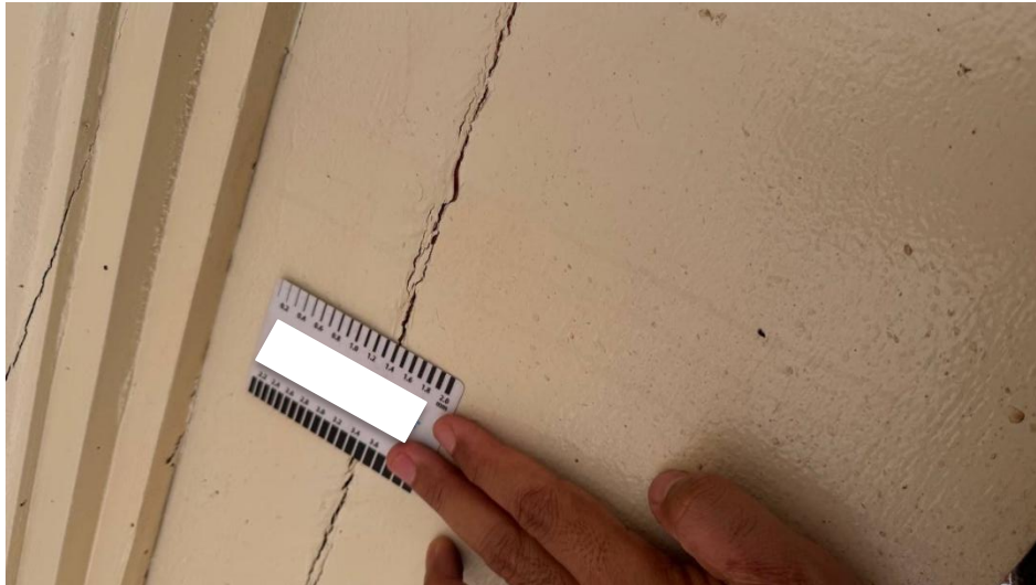
Fig 2. The process of measuring crack width with a measuring device
