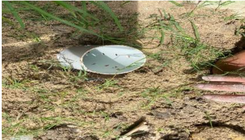
Gambar 4. Penanaman pipa biopori ke lubang
