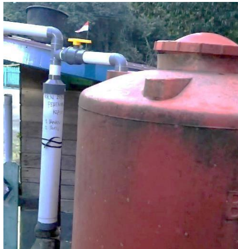
Gambar 6. Sistem Rain Water Harvesting RT. 23 Dusun Mekar Baru
